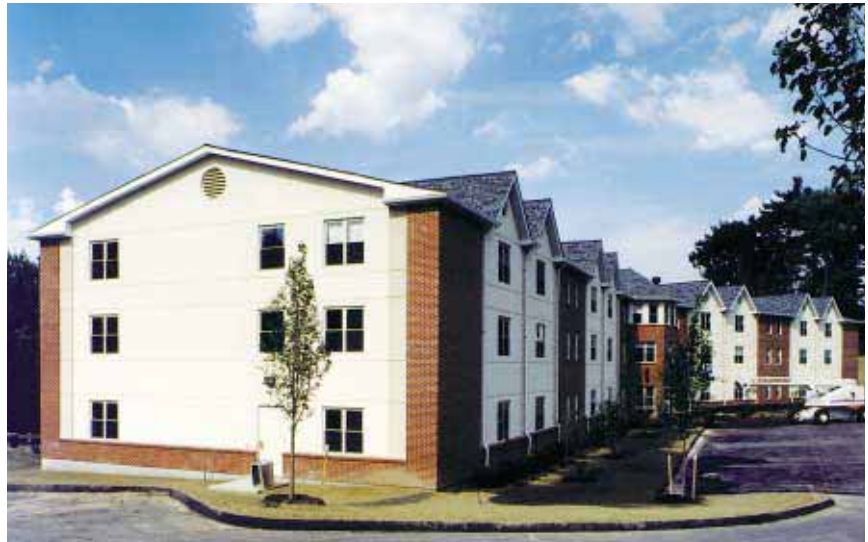
The finished dormitory at Curry College houses 148 students in a residential setting. Architect George Dakin notes that architectural panels could easily be combined with hollowcore floors and ceilings to fit into the context of surrounding buildings at a college or university.
